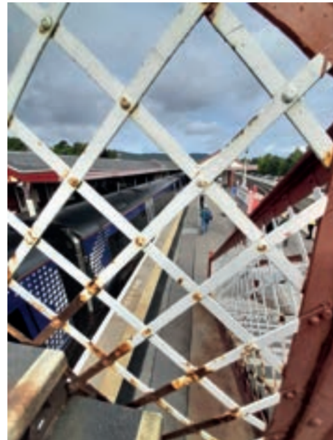
The diamond pattern shown on this station bridge has also inspire my costume design.
